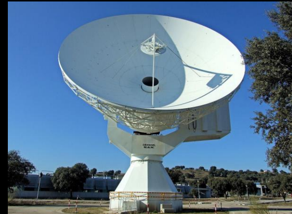
15m satellite tracking antenna at ESA's European Space Astronomy Centre (ESAC) converted into a radio telescope
